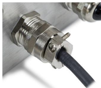
Figure 2-74: Cable Gland Installed
